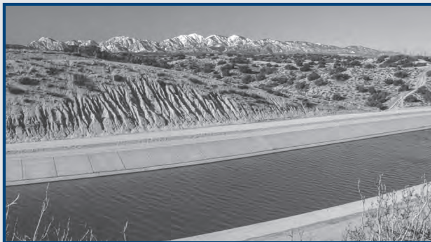
A State Water Project canal with snow covered mountains.
