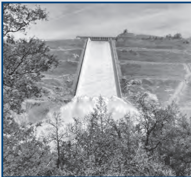
Oroville Dam Spilling on the State Water Project.
